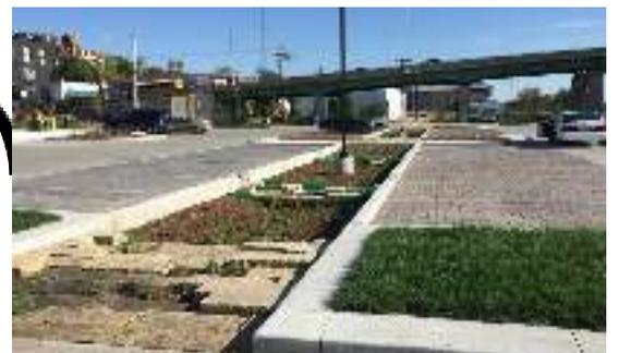
*Permeable Pavers & Bioretention Cells
