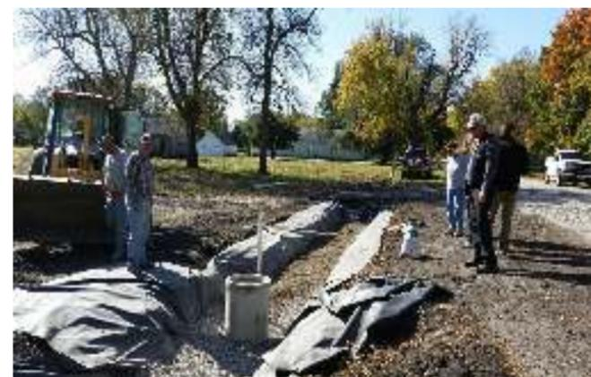
Bioretention cell being installed in Lohrville
