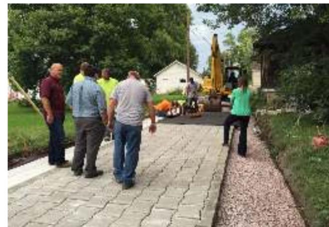
Permeable paver alley being installed in Kingsley
