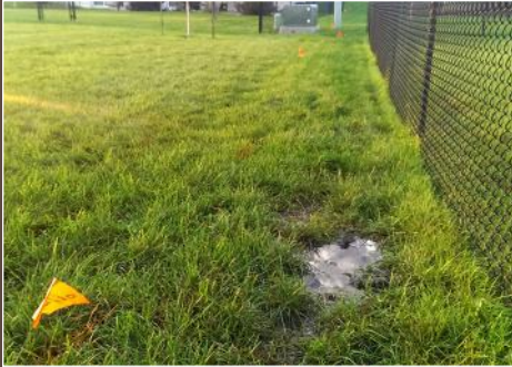
Lack of water infiltration
