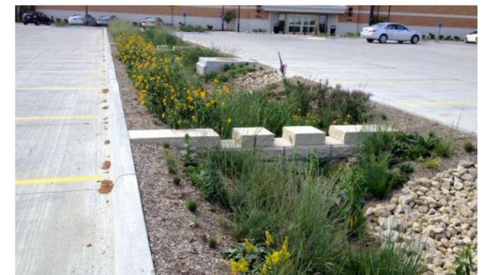
Stormwater runs off large parking lots very quickly. Bioswales are a great way to capture and infiltrate runoff from small events. Large events are conveyed to a storm sewer intake at the bottom of this swale. This bioswale provides an aesthetically pleasing green space in this Coralville parking lot.
