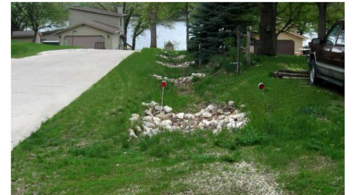
A newly completed bioswale with rock checks in a road ditch above East Okoboji Lake reduces runoff and sediment that used to be delivered to the lake with each runoff event. Rock checks help hold and infiltrate stormwater.
